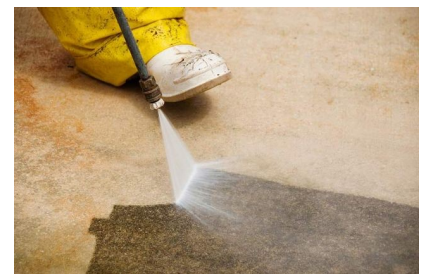
Water blasting of roofs and sidewalks.
